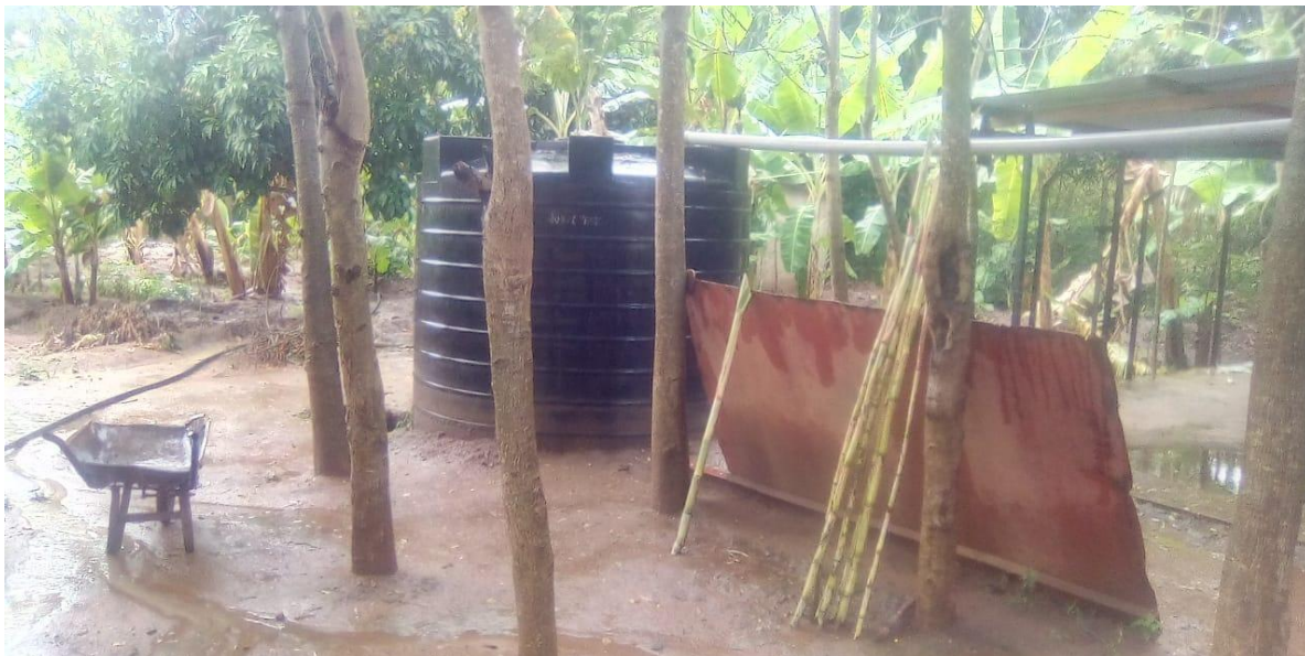
Figure 8: A water tank collecting water at FOM Offices roof
